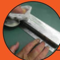
3. Ensure surfaces have fully dried following final clean down before applying the tape to the first surface ensuring correct positioning.
